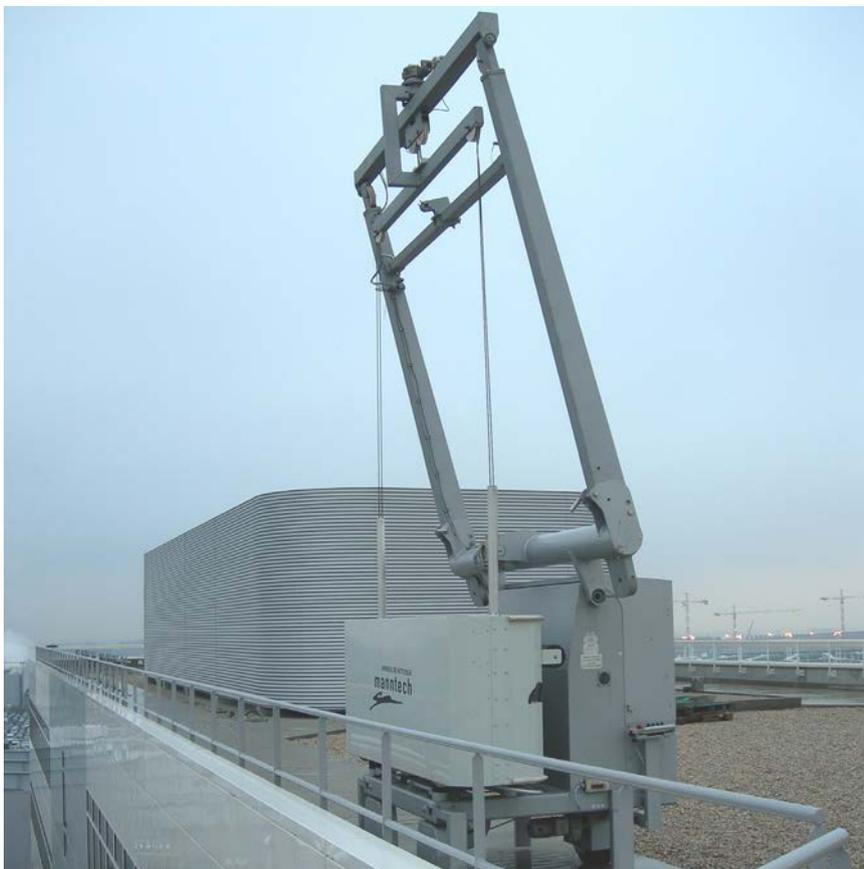
Type 1.3 with crossbar for load-bearing hoist
