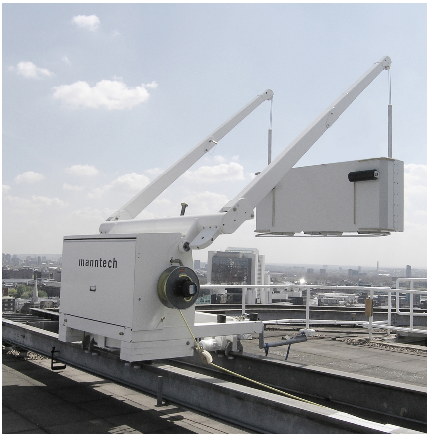
Type 1.1 with retractable jibs for parked position
