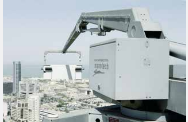
Type 6.1 track-based with vertical slewing articulated jib to reach recessed building areas
